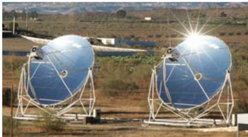
*Figure 5.* Dish/Stirling System at PSA (Almería/Spain)
